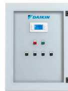
(Light/Full) (≤4/≤8 MT3 chillers & peripherals)
