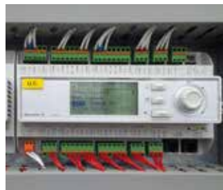
Controller box upgrade
